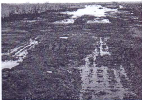
Fig D: picture taken after backfilled
